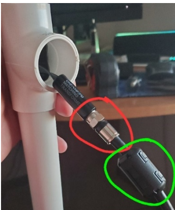
Figure 11 - Coax attached to Transformer with Choke installed
